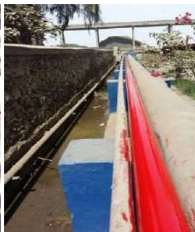
WRAPPING COATING ON FIRE PIPELINES AT ULTRATECH CEMENT KOVAYA
