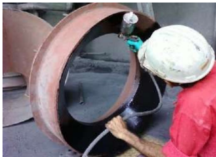
INNER CERAMIC COATING ON T-BEND COATING ON VENTURY OF BOILERS SEA WATER PIPE
