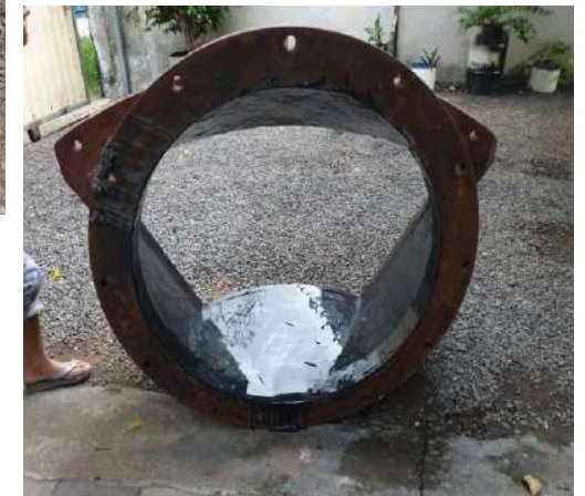
CERAMIC COATING APPLIED ON INNER SUFACE OF COOLING TOWER SEA WATER PIPES
