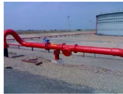
WRAPPING COATING ON FIRE PIPELINES AT ESSAR OIL JAMNAGAR
