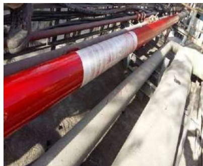
WRAPPING COATING ON FIRE PIPELINES AT ULTRATECH CEMENT KOVAYA
