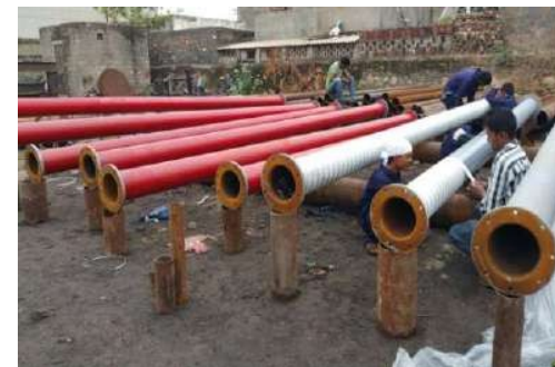
WRAPPING COATING ON FIRE PIPELINES AT TATA CHEMICALS MITHAPUR
