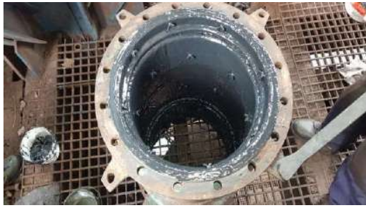
INNER CERAMIC COATING ON T-BEND COATING ON VENTURY OF BOILERS SEA WATER PIPE
