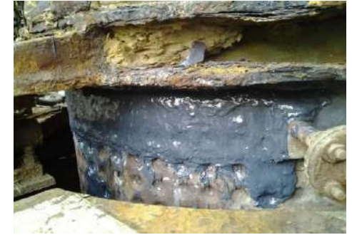
HCFC PLANT REACTOR JACKET
