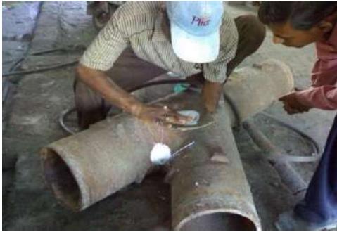
LEAKAGE SEALED ON JOINTED PIPES
