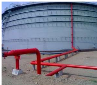
WRAPPING COATING ON FIRE PIPELINES AT ESSAR OIL JAMNAGAR
